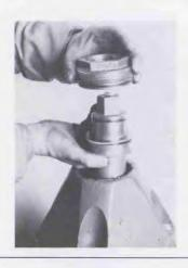
2 Remove operating nut (1) by rotating C.C.W. on O.L. hydrants, C.W. on O.R. Hydrants.
