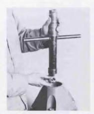
3 Insert unthreaded end of hydrant wrench combination tool over stem and lower into hydrant until socket engages hex stop nut (12). Unthread and remove nut by turning in same direction as operating nut in Step 2.
