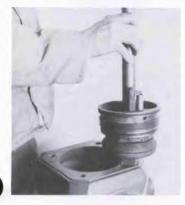
Valve assembly can now be lifted out of hydrant.
