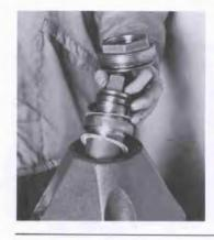
Before commencing disassembly procedure, shut off water in main controlling flow to hydrant inlet.
