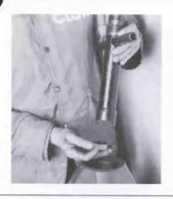
Insert unthreaded end of hydrant wrench combination tool over stem and lower into hydrant until socket engages hex stop nut (12). Unscrew and remove nut by turning in the same direction as operating nut in Step 3.
