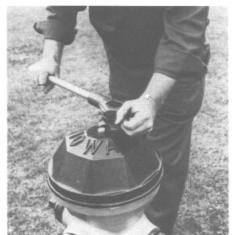
Close hydrant valve, open valve in the main controlling flow to the hydrant.
