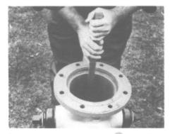
Grasp square operating rod 20 and lift to remove working parts from hydrant barrel. Note position of all parts before disturbing
