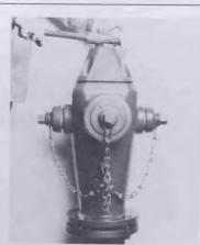
Open hydrant to test joints for leaks.
