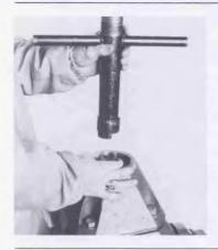
3 Insert unthreaded end of hydrant wrench combination tool over stem and lower into hydrant until socket engages hex stop nut (12). Unthread and remove nut by turning in same direction as operating nut in step 2. Lower portion of stem must be held with a pipe wrench or other means to keep from turning. Pull upper stem out of cover.
