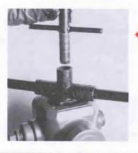
Slowly rotate clockwise until threads engage, then rotate approximately six full turns and tighten securely. Tightening torque must be at least 100 ft-lbs, but should not exceed 150 ft-lbs. Remove combination tool and hydrant wrench from upper stem.
