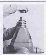
20 Screw operating nut (1) onto upper stem with one Delrin bearing (42) in place. Install remaining Delrin bearing (42) between two races (5) on operating nut.
