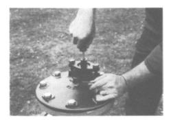
Replace complete head assembly 11 over operating rod 20 and bolt to standpipe 19 in original position. Unscrew bronze cap screw 4 from 5, insert screwdriver and turn adjusting screw 10 down against top of operating rod 20, then back off one-half turn. Replace cap screw 4. Examine packing 8 and replace if necessary.
