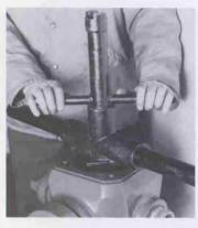
6 Lower hydrant wrench over stem. Insert threaded end of combination tool into top of hydrant wrench and thread it onto stem. Tighten combination tool stem until hydrant is pulled into closed position.
