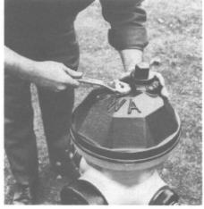
Replace hydrant dome 2, tighten bolt 3
