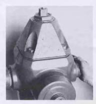
11 To test drain valve, remove one hose nozzle cap and open hydrant five turns. Allow water to rise to level of nozzle. Close hydrant and place hand over nozzle opening. Suction should be felt which indicates drain is working properly.
