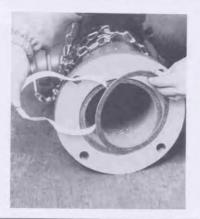
5 Clean top surface of standpipe (6) remove adhesive backing on new gasket (51) and insert into recess in bottom of nozzle section.
