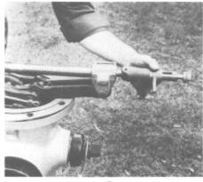
Unscrew lifter guide 43 to attain full open position of the drain valve assembly, then turn guide back one full turn. Adjust to position it in line with the assembly
