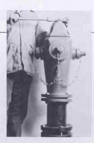
Open hydrant to test joints for leaks.
