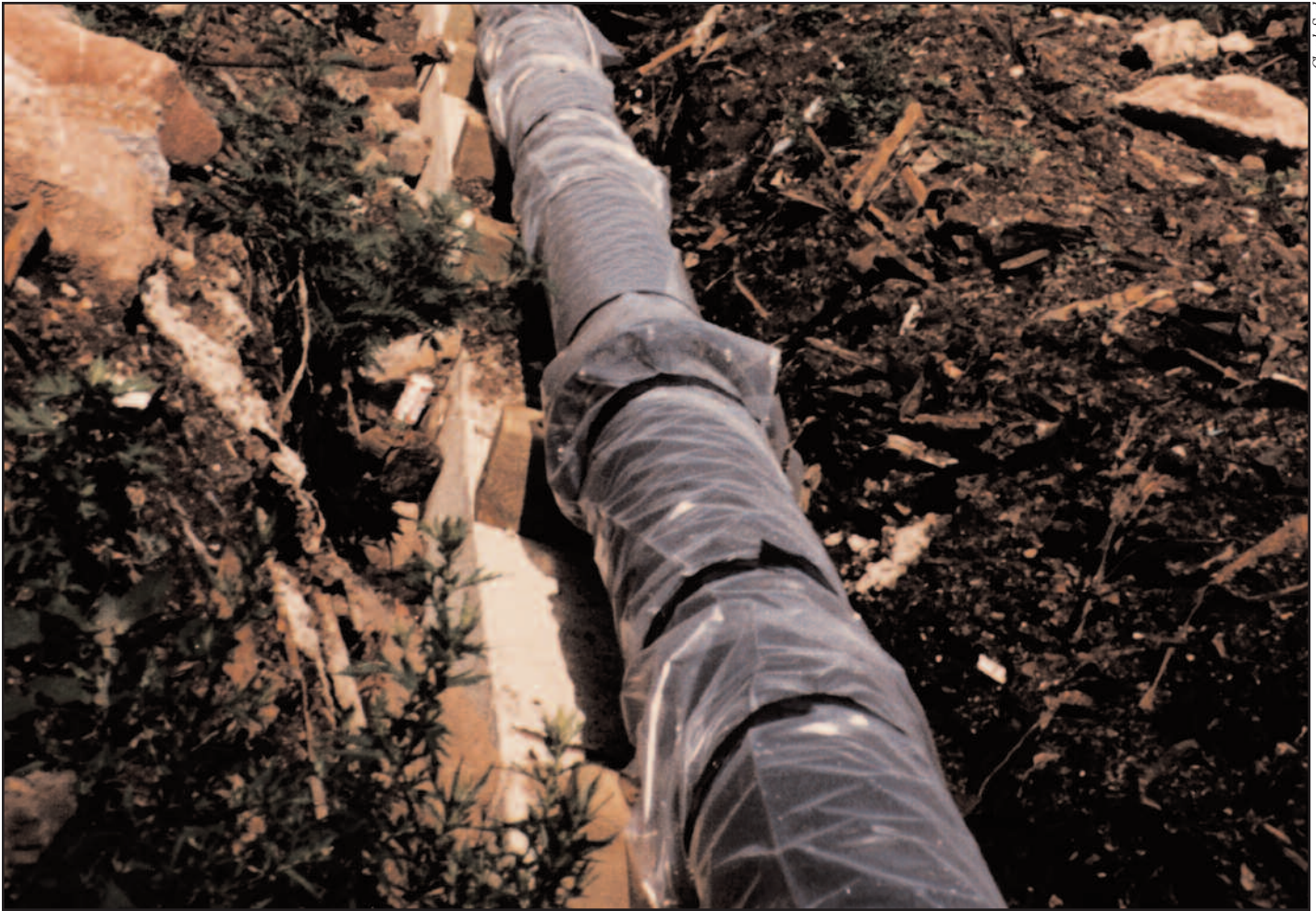
Although most soil environments are not considered corrosive to Ductile Iron pipe, soils in landfill sites such as the one pictured here are generally considered corrosive. Other typically corrosive environments include swamps, peat bogs, expansive clays, and alkali soils.
