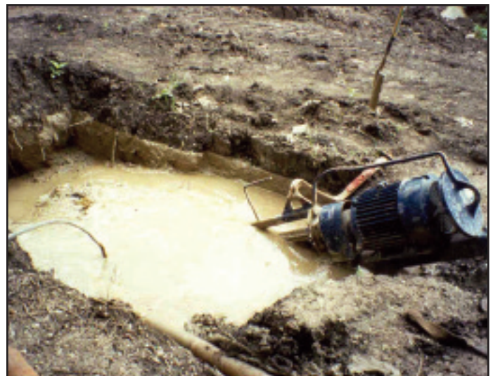
HDD Entrance Pit and Drilling Mud Recycling Pump
